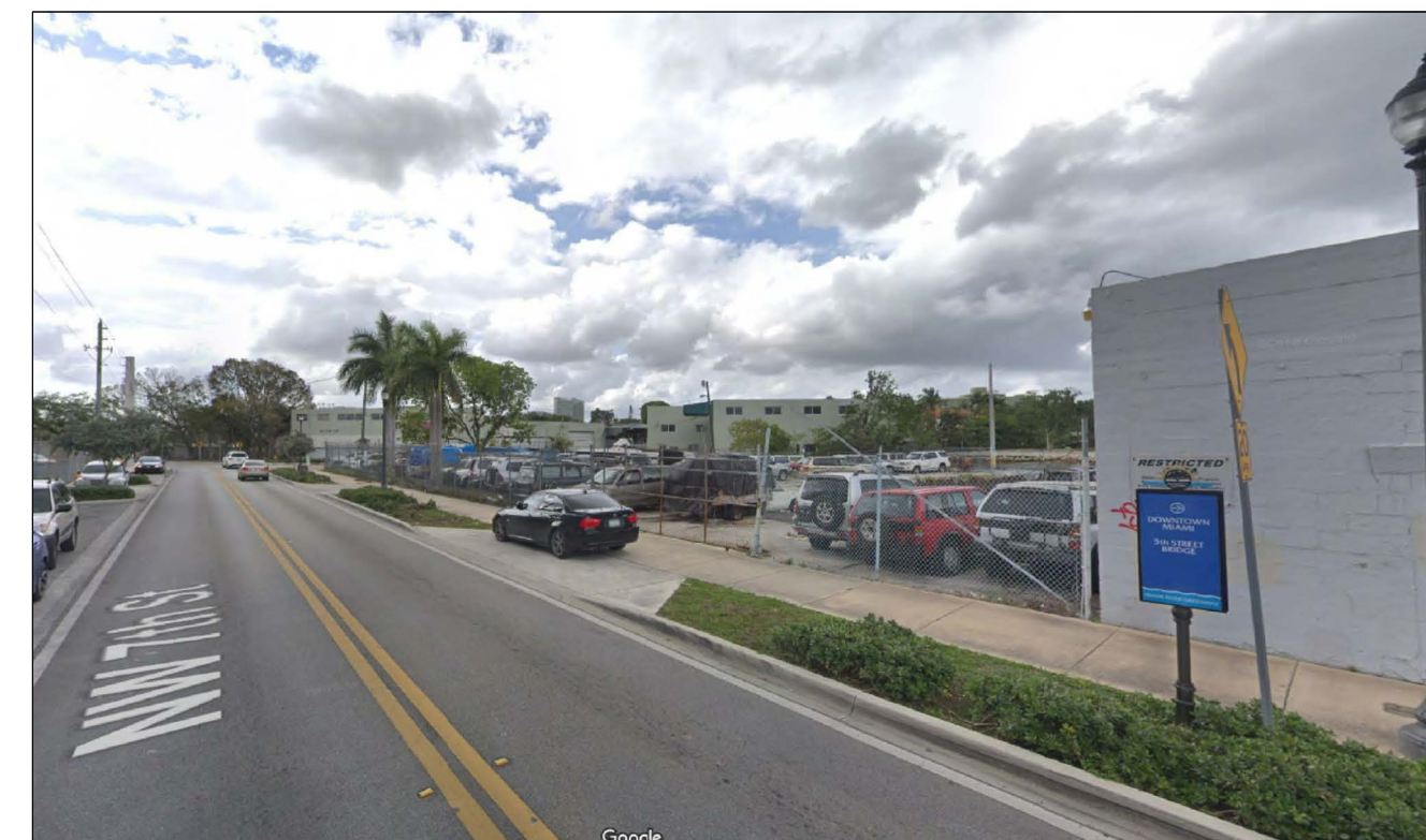
(1) 0 FT EXISTING BUILDING (555 NW S RIVER DR.)
