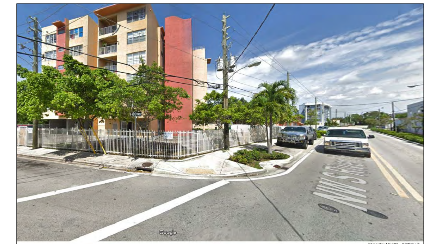
(8) 0 FT EXISTING FENCE (437 NW S RIVER DR.)
