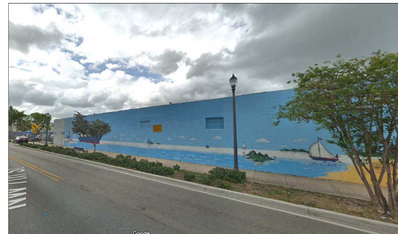
(2) 0 FT EXISTING WALL (631 NW S RIVER DR.)
