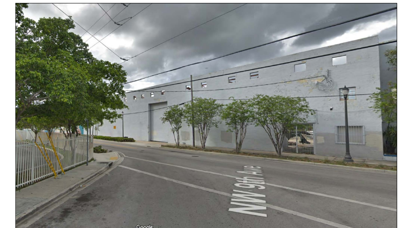
(4) 0 FT EXISTING FENCE (936 NW S RIVER DR.)
